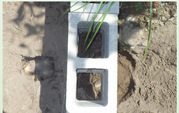
A 14-pound Sulcata dug this hole on the right side of the wall and extended it underneath and past, causing eventual collapse of the wall.
